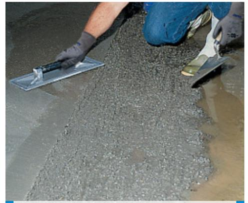
Screeding with mortar admixed with Idrosilex Liquid
