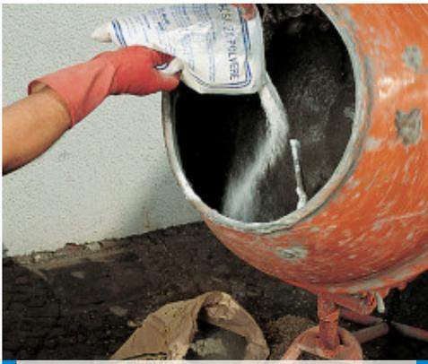
Preparing waterproof mortar admixed with Idrosilex Powder
